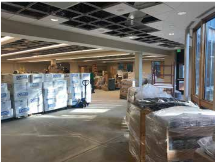
The Collection Area, with CDs wrapped on the right and windows looking out to the Literary Garden
