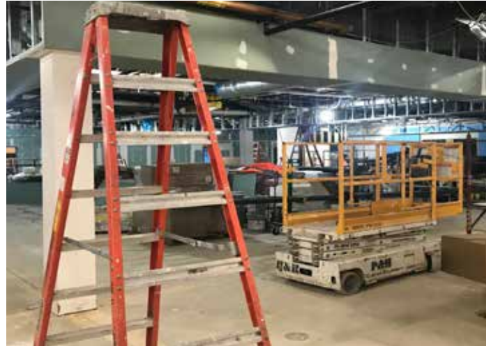
Current state of the Collection and Reading Room areas
