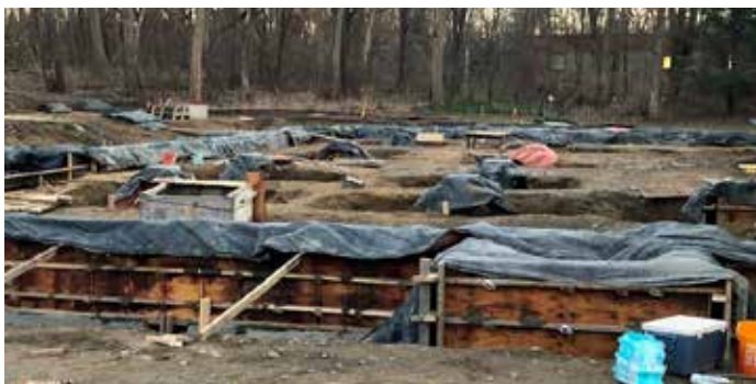
Building the foundation for the new children's addition
